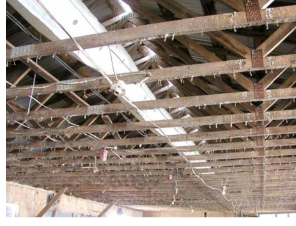
Figure 7. Air tube installed within truss structure to reduce impact of wind.
