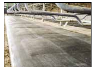
Renovation of the damaged mattresses with Aquatop
