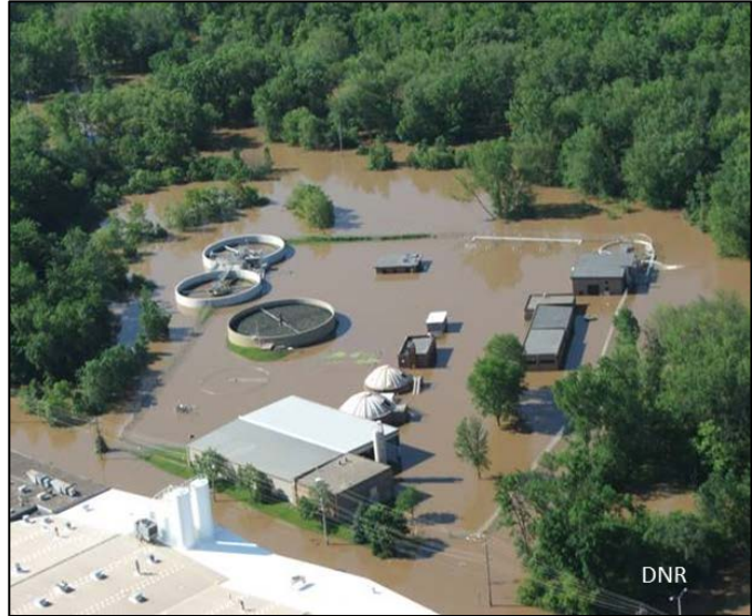
Reedsburg Wastewater Plant inundated with floodwater, June 2008
