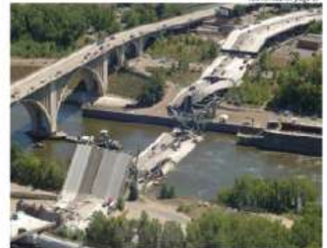
At the north end of the bridge and looking towards the south.
