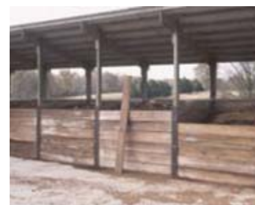
Figure 5: A typical compost bin, which requires the lifting of heavy boards to place dead birds within.
